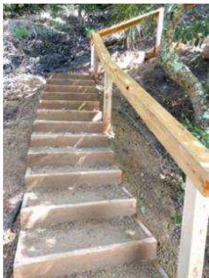
Image 33. : Stair build Lake Tyers Beach
