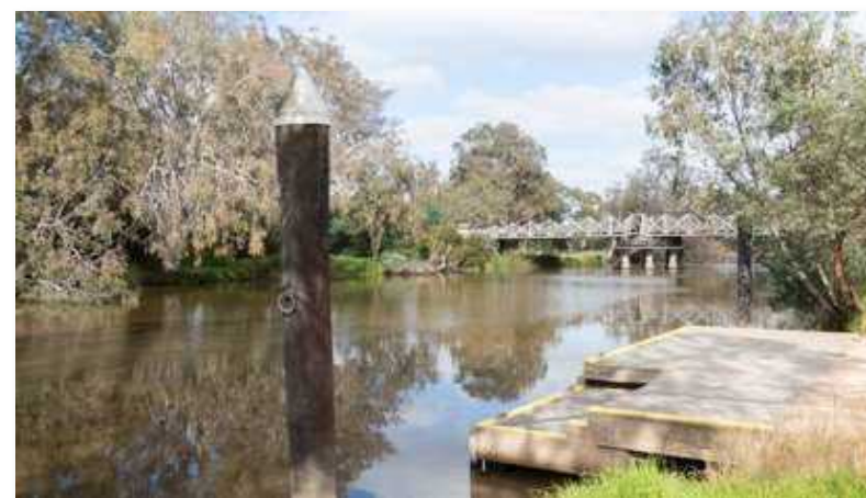
Image 60. Static jetty, historic swingbridge, Latrobe River
