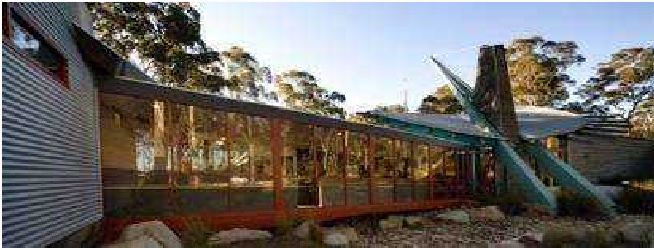
Image 48. Existing Gunaikurnai Cultural centre
