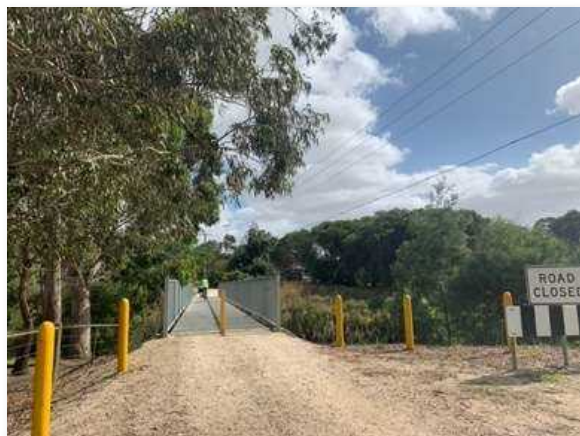
Image 37. IMAGE: existing bridge near Sale township
