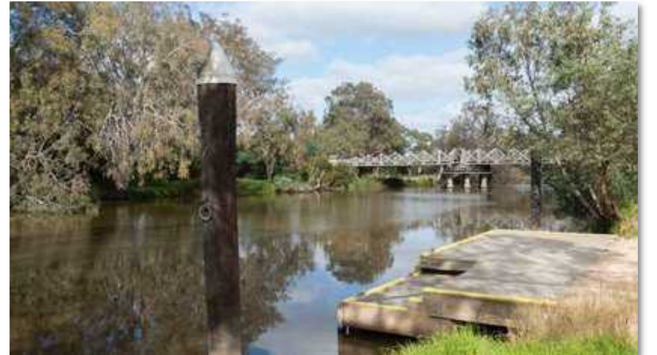
Image 54. Existing boat jetty platform located eastern side of historical swingbridge, Latrobe River
