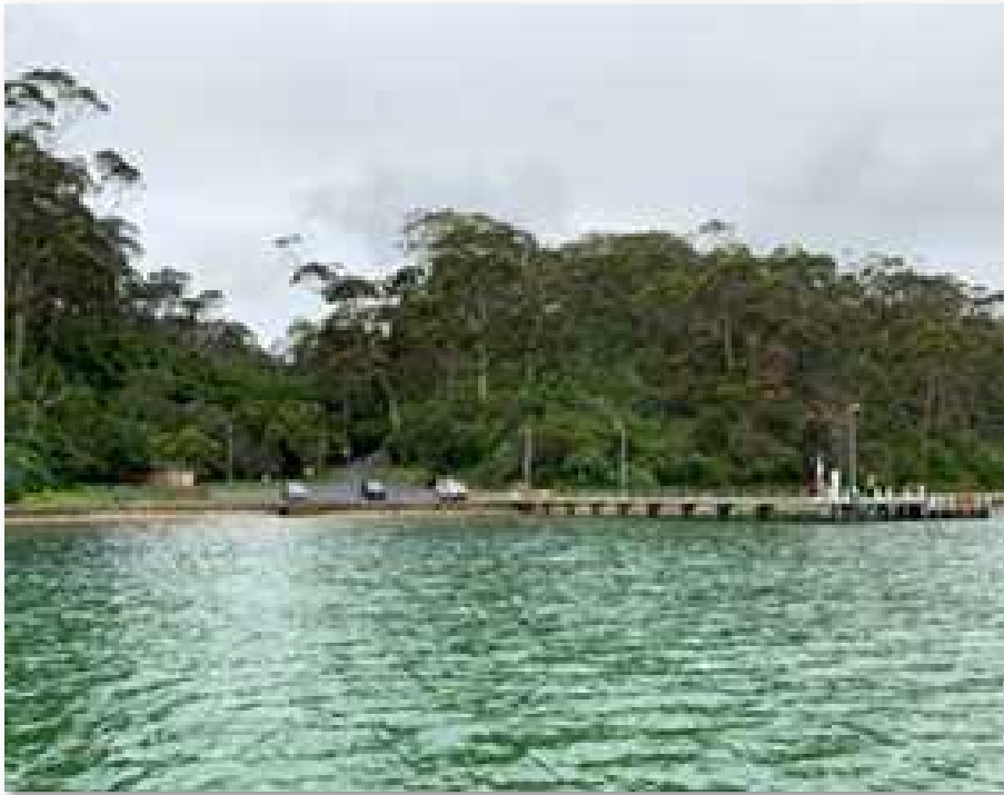
Image 16. Kalimna Jetty. Existing rock wall walkway to east (frame right).
