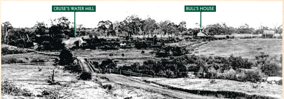
Ellen's Brook at Belhus photographed in May 1866 showing the bridge and road built by convicts and Aboriginal prisoners. William Cruse's watermill built in April 1837, visible at the end of the bridge, ground wheat into flour. The road and part of the original bridge are still present.
