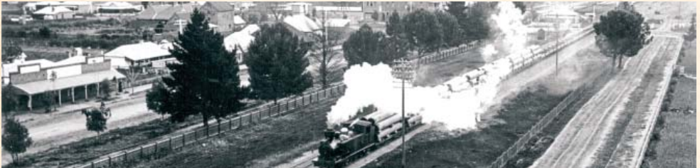
A train on the new dual track rail carrying pipes for the Goldfields Water Supply Scheme photographed from the Post Office tower c1900. Courtesy State Library of Western Australia 1797B
